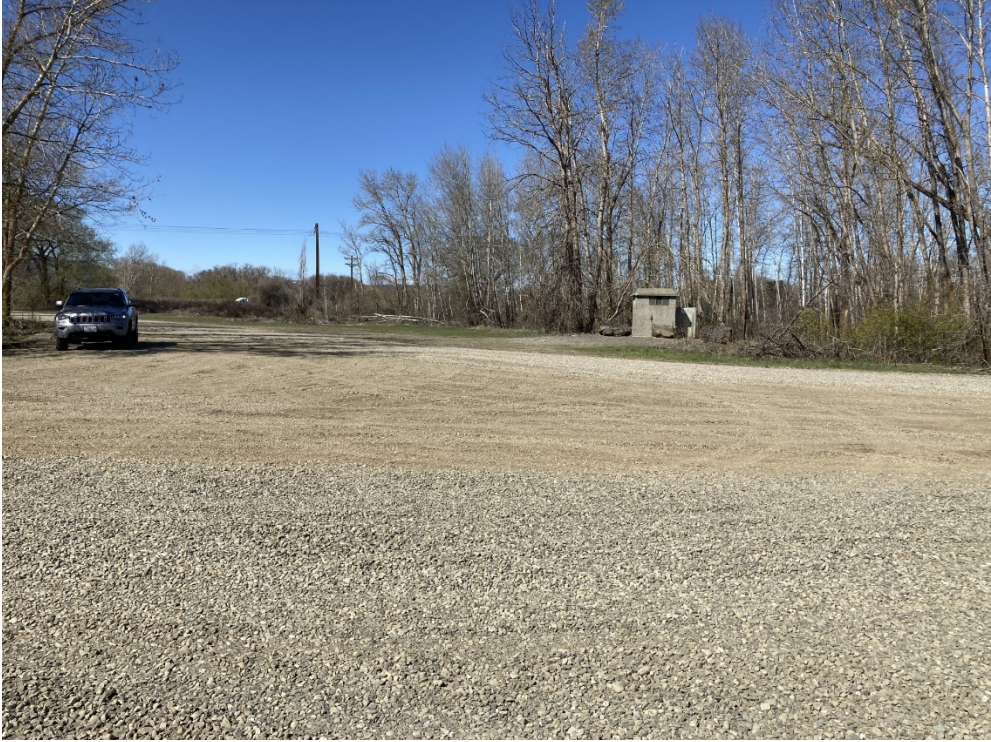
Photo 2. Existing parking lot and vault toilet, both to be regraded/replaced
